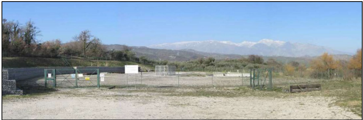
Colle Santo Well Site
